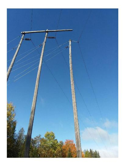
Three pole light angle wood pole structure - top of right pole burned off by lightning strike, middle pole rejected due to insufficient shell strength caused by internal decay/rot
