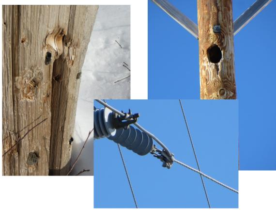
Rotting pole bases resulting in a leaning pole, other poles with cracked base and woodpecker damage, small 3/0 ACSR conductor
