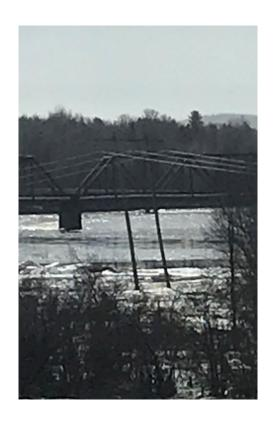
2019 spring flooding impacted structures alongside Salmon **Brook destabilizing** them and conductor too low for navigable waterway. Rebuild to include taller heavier class composite poles placed on berms with culverts and stone backfill.
