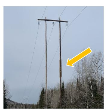
Woodpeckers nesting activity has damaged many poles while others need to be replaced because of wood pole failure
